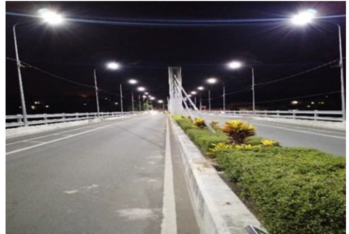
a) Bridge of Progress, Batangas City.
