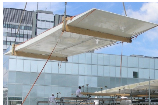
Figure 11. Lightweight GFRP sandwich roof [24]
