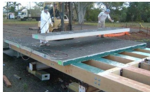
Figure 8. FRP sandwich bridge beams at USQ
