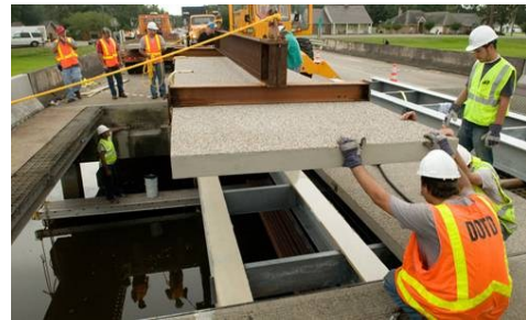
Figure 4. Balsa-cored composite bridge deck [13]
